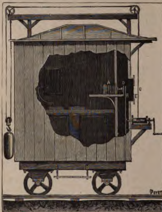
FIG. 7.—INTERIOR ARRANGEMENT OF THE DARK CHAMBER.
